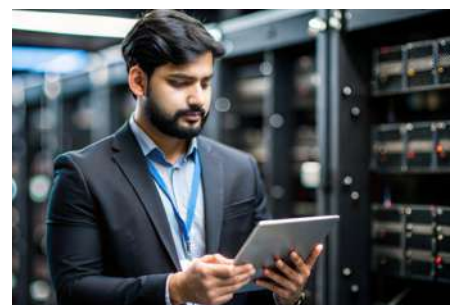
Mini Datacenters, Server Rooms & Battery Rooms
